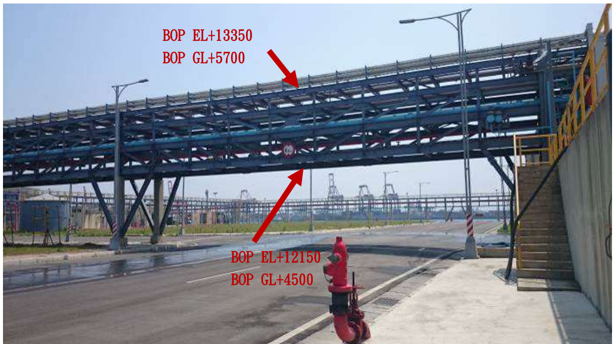
施工前 103.5.14 1. BOP GL+5700 2. BOP GL+4500 1. BOP EL+13350 2. BOP EL+12150
